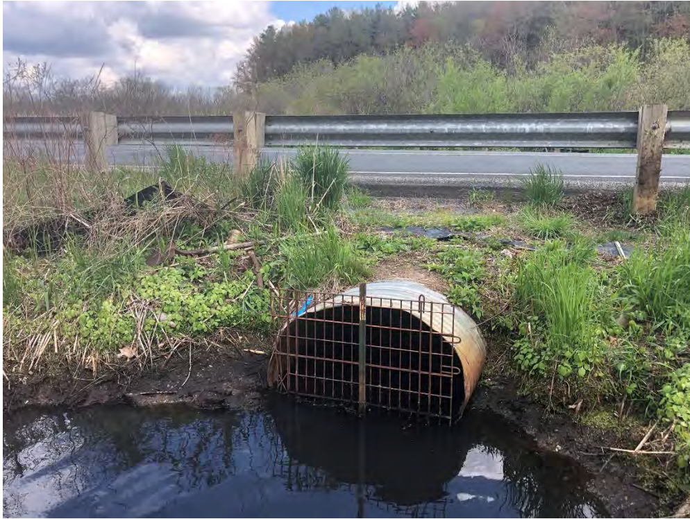
Photo 27. Monitoring Site 7 facing east
