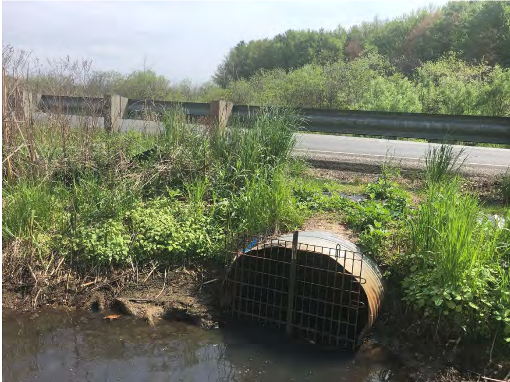
Photo 27. Monitoring Site 7 facing east
